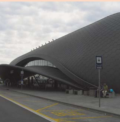
Airport, Brno, Czech republic
